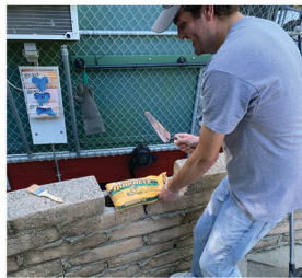
Kevin Fixes the Wall
